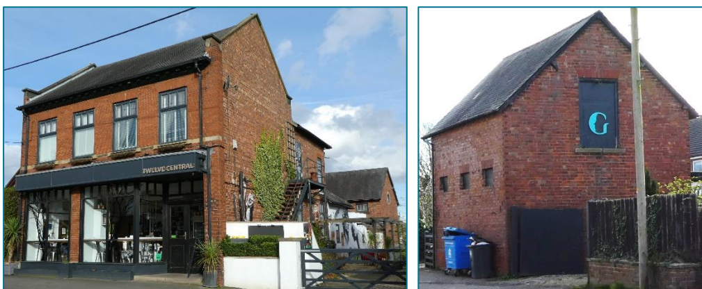
Left: Former [L] Co-op along Middleton Lane with detached Stable building in the background. Right: Stable viewed from Yarm Road. (Photos © Gaby Rose, March 2024)
