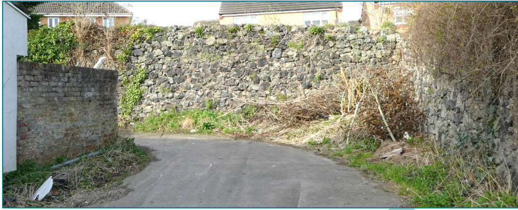
Top: Remains of southern boundary wall of the [N] Middleton Iron Works, bordering the back lane to Killinghall Row, Yarm Road, the first houses to be built for the increasing workforce. The wall seems to be constructed from rubble limestone, which is an untypical construction material for the area. Limestone was brought in from Weardale and used for forming the slag in smelting 87 . (Photo © Gaby Rose, March 2024)
