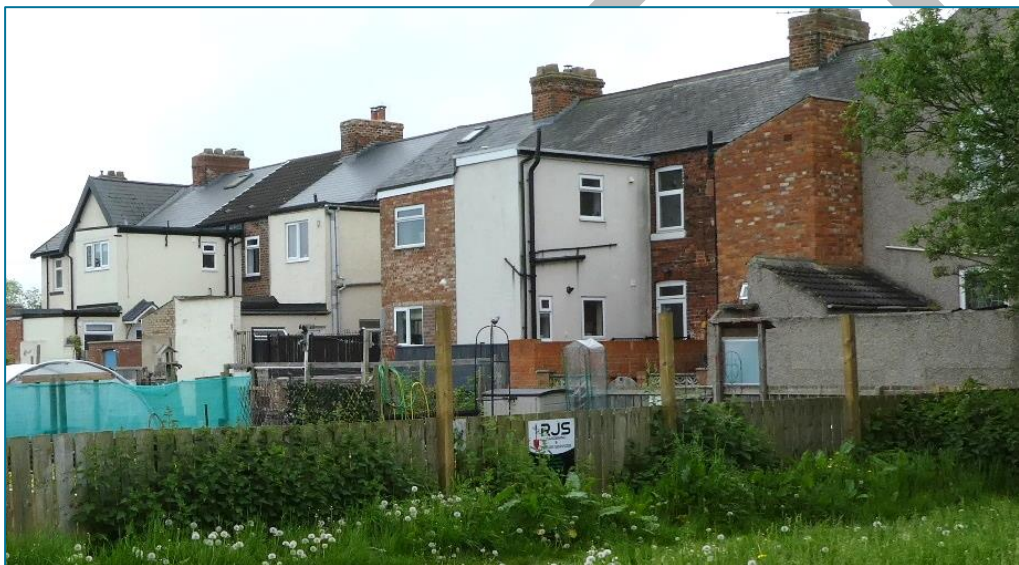
Extensions to rear of traditional terrace with flat roofs, modern renders and inappropriate window proportions, viewed from public footpath. (Photo © Gaby Rose, May 2024)
