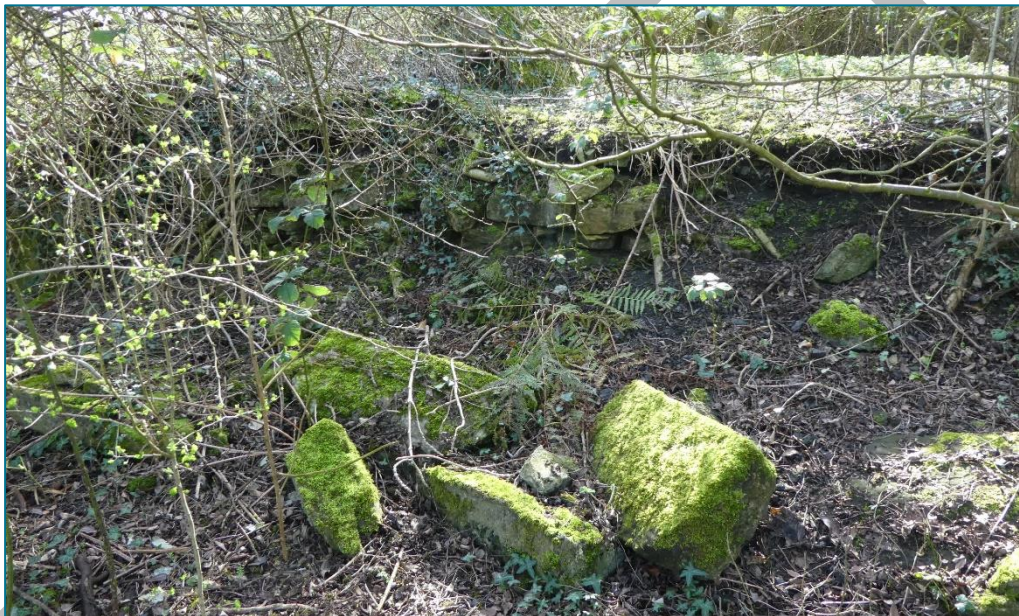
[A] Crane Base (top) and Platform (bottom). Top : Looking northwest, the platform is behind the crane base within the undergrowth; its alignment shown on the 1913 map is indicated by the yellow line. The rail tracks coming from the main railway line would have been to the righthand side. Bottom : Remnants of former platform viewed from the bridlepath looking southwest, with the walling stones now largely dislodged. The crane base is to the left just outside the view. (Photos © Gaby Rose, March 2024)
